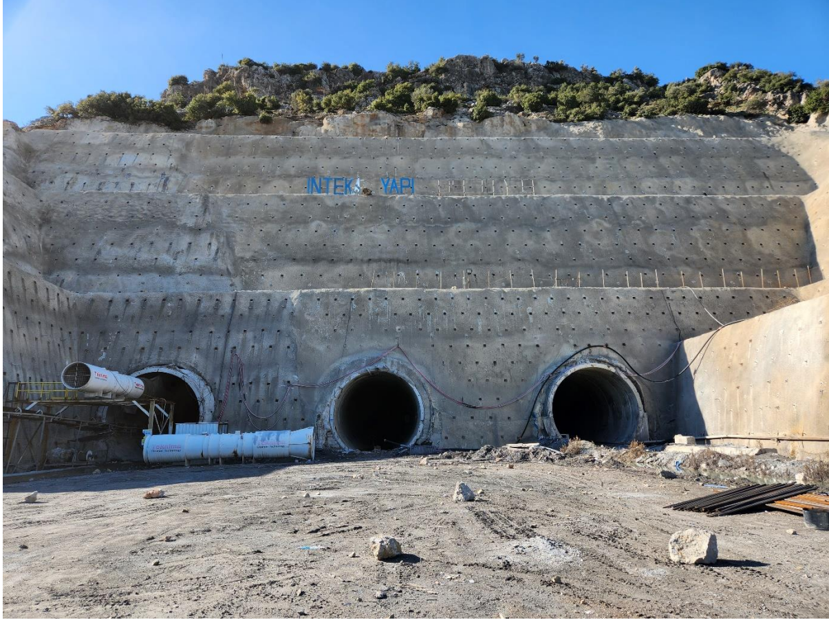
Figure 6.10. Nurdağı portal of Bahçe-Nurdağı railway tunnels
