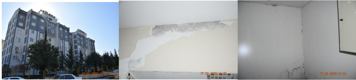
Figure 5.5. Performance of a tunnel form building
