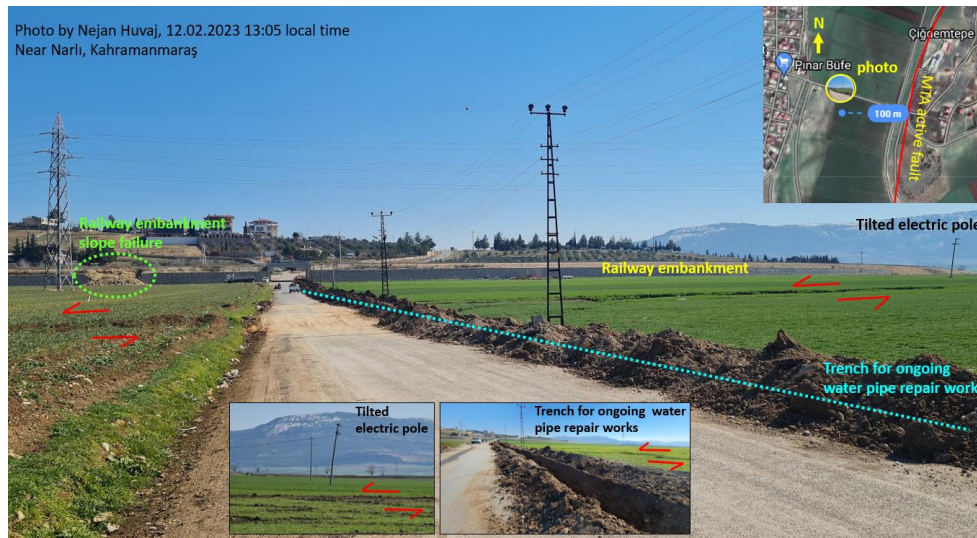
Figure 8.3. Referring to Figure 2 for locations of the photos: offset on the road due to surface fault rupture, railway embankment slope instability, water pipeline repair works and a tilted electric pole can be seen, near Narlı, Kahramanmaraş. (Active fault data is taken from Emre et al. (2013) published by the General Directorate of Mineral Research and Exploration, MTA (Maden Tetkik ve Arama Genel Müdürlüğü)).
