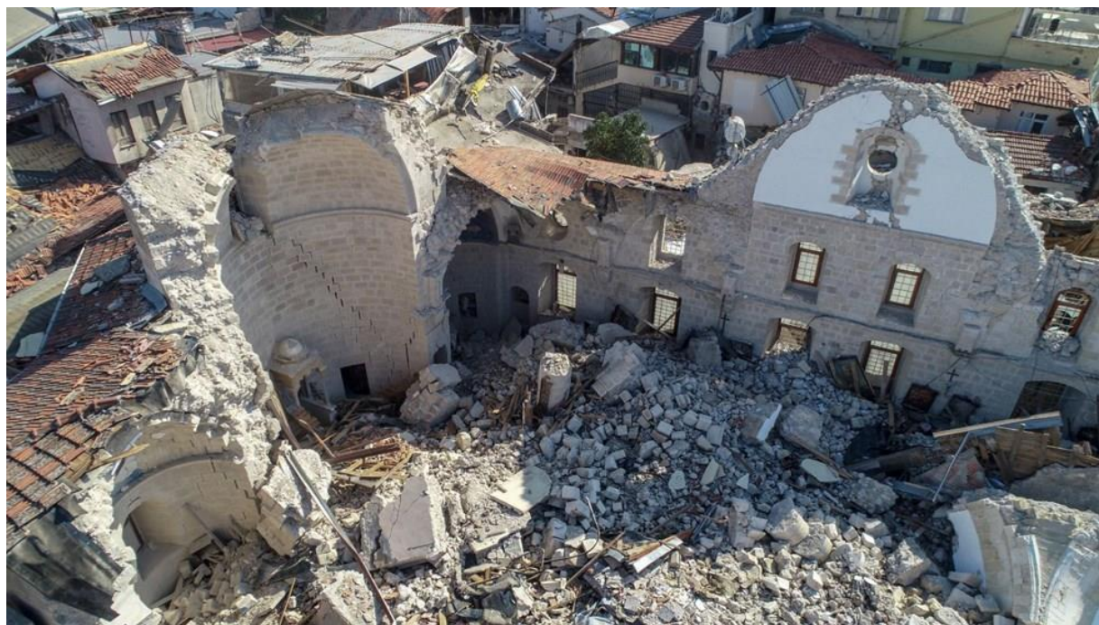
Figure 9.7. The Antakya Rum Protestant Church after the earthquake
