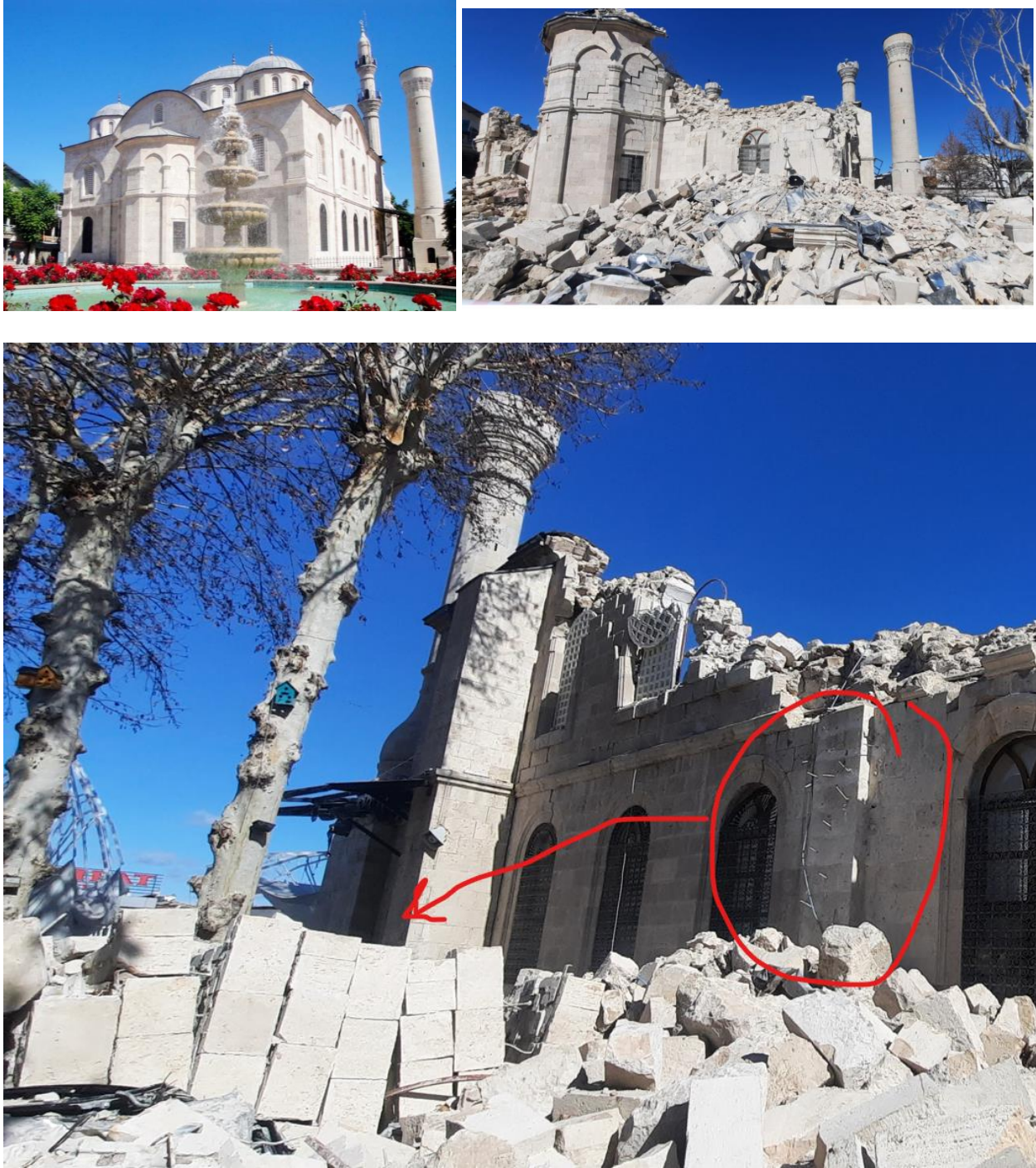
Figure 9.4. Yeni Cami (new mosque) before and after pictures and short anchorage.
