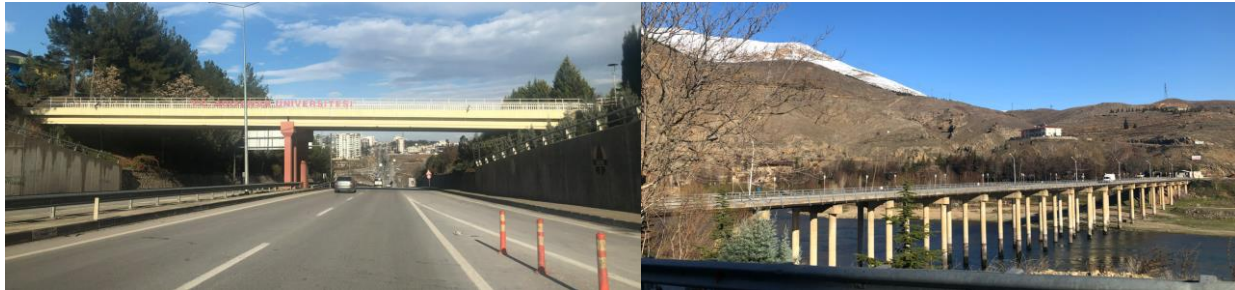
Figure 6.8. Bridge typical have no damage
