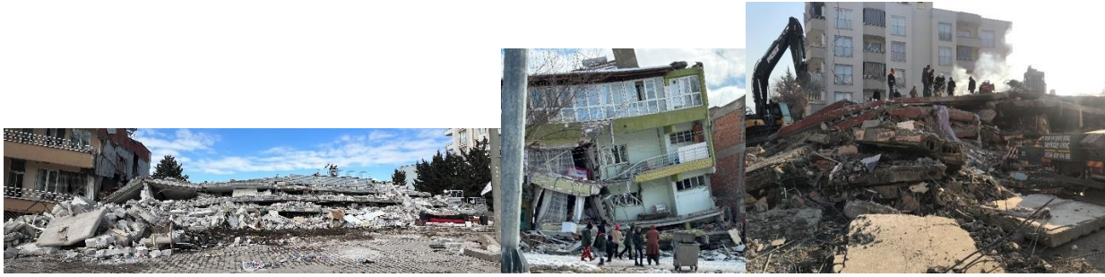
Figure 5.2. Building Collapse in Malatya
