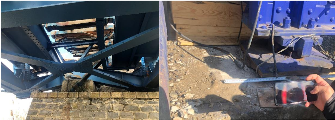
Figure 6.4. Bearing dislocation and movement
