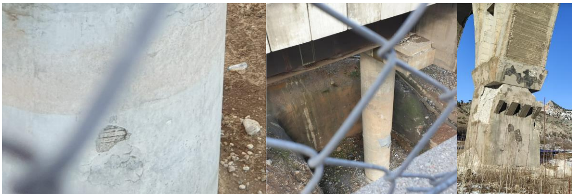
Figure 6.3. Concrete spalling
