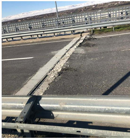
Figure 6.1. Abutment rotation due to seismic soil liquefaction induced foundation failure
