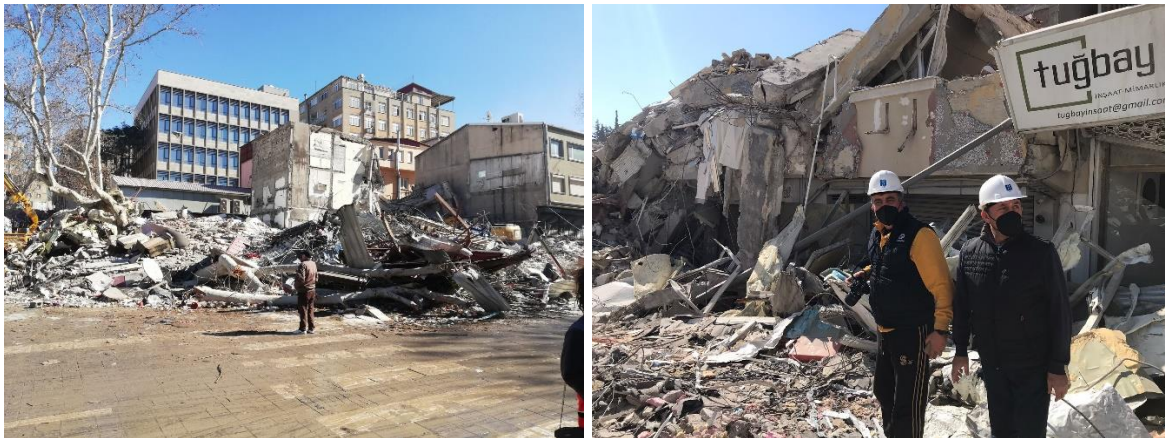
Figure 5.1. Building Collapse in Antakya and Kahramanmaraş
