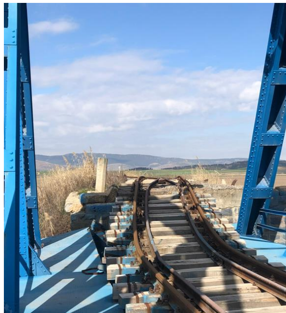
Figure 6.4. Bearing dislocation and movement
