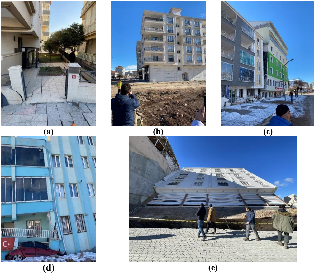
Figure 4.4. Poor foundation performance in a) Çay District / İskenderun / Hatay ( 36.5911^{\circ}N , 36.1790^{\circ}E ), b) Hürriyet District / Gölbaşı / Adıyaman ( 37.778^{\circ}N 37.628^{\circ}E ), c) Yavuz Selim District / Gölbaşı / Adıyaman ( 37.788^{\circ}N , 37.642^{\circ}E ), d) Yavuz Selim District / Gölbaşı / Adıyaman ( 37.788^{\circ}N , 37.642^{\circ}E ), e) Yavuz Selim District / Gölbaşı / Adıyaman ( 37.78827^{\circ}N 37.64879^{\circ}E )
